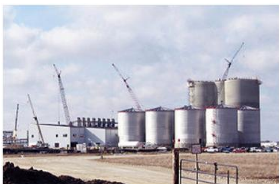
Figure 1 An ethanol fuel plant under construction, Butler County, Iowa
